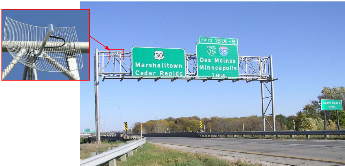
Figure 3-9. Wireless communication equipment installed at the west end of the bridge.
