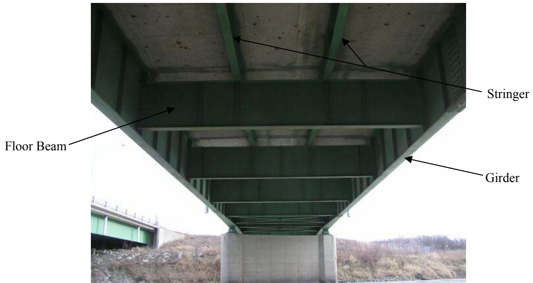
(c) Bottom view (looking east)
