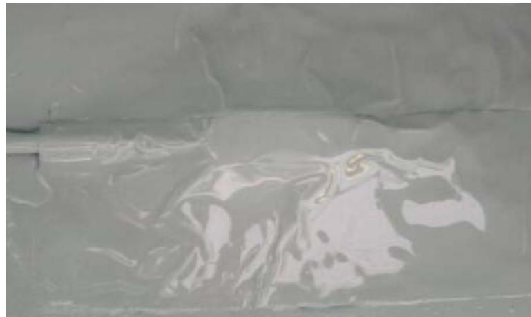
(c) Strain gage protected with butyl rubber underneath aluminum foil tape and primer
