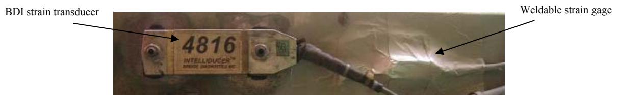
(b) BDI strain transducer installed next to the weldable strain gage
